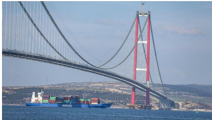
Figure 2: The Strait of Çanakkale and 1915 Çanakkale Bridge [10]
