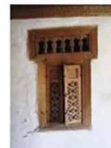
Figure 10. Ventilation elements in the walls above windows [27]
