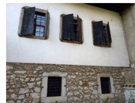
Figure 7. Iron window shutters on windows (Authors, 2022)
